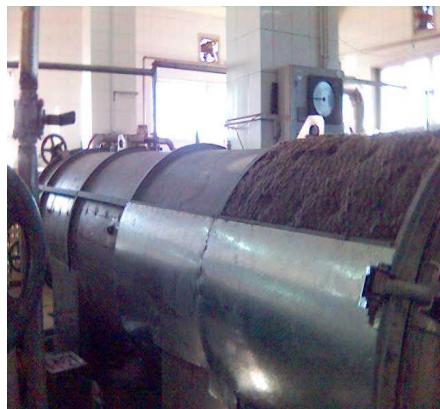
Insulation of sterilizer using rock wool and aluminium foil (implemented CP measure)
